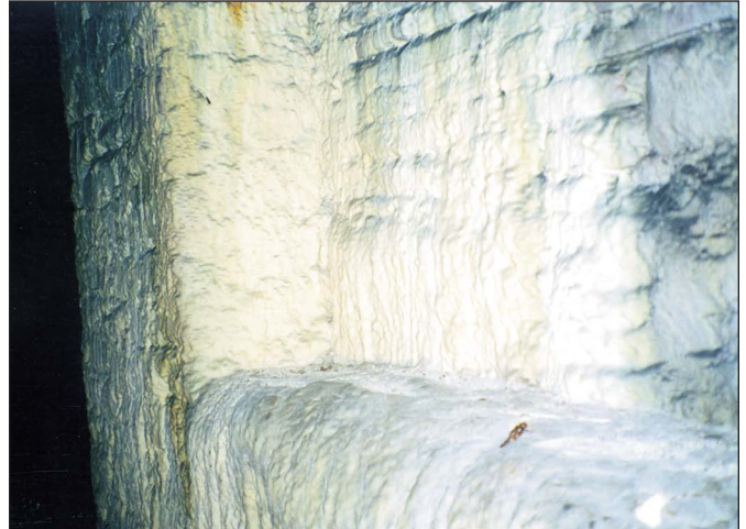
Figure 37. Detail of pier, inner ledge below L1. (Photo: J. Dello Russo)
