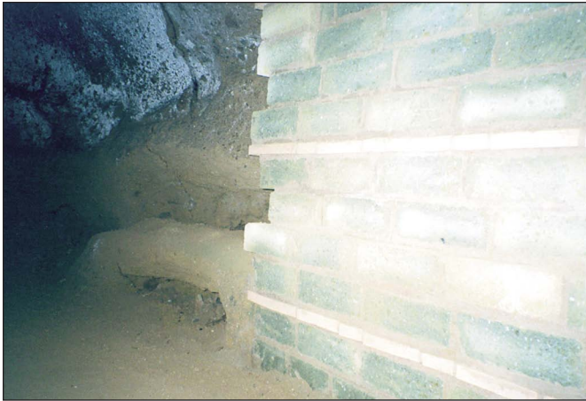
Figure 48. Restored wall in E1, just beyond lucernarium L2. (Photo: J. Dello Russo)
