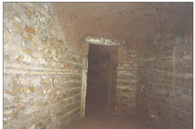
Figure 26. Doorway into catacomb proper, raised in late twentieth century to present height (Photo: J. Dello Russo)
