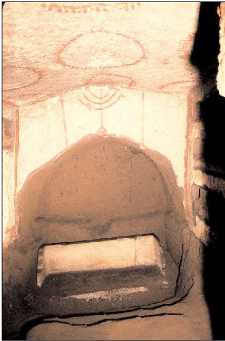
Figure 50. Interior of cubiculum Gb, prior to repairs made to floor and right wall. (Photo: Estelle S. Brettman, ICS photo archive)
