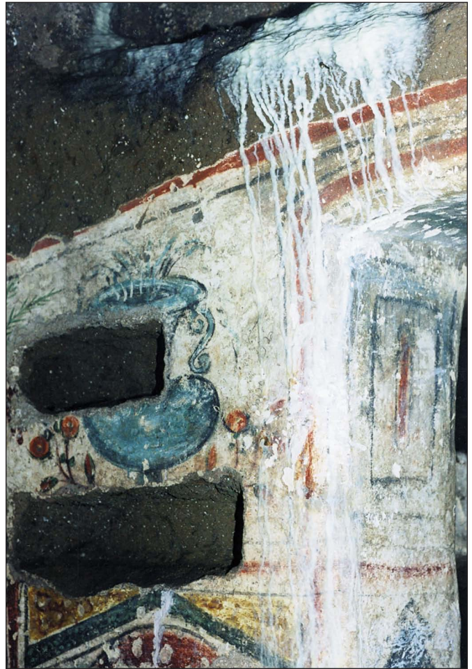
Figure 28. Interior of cubiculum Da, walls around door and ceiling damaged by the addition of later tombs (Photo: J. Dello Russo).
