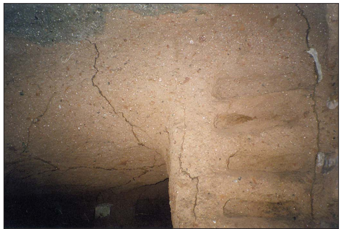
Figure 57. Heightened gallery level in G1 at its intersection with G1b: detail of children's loculi on narrow pier. (Photo: J. Dello Russo)
