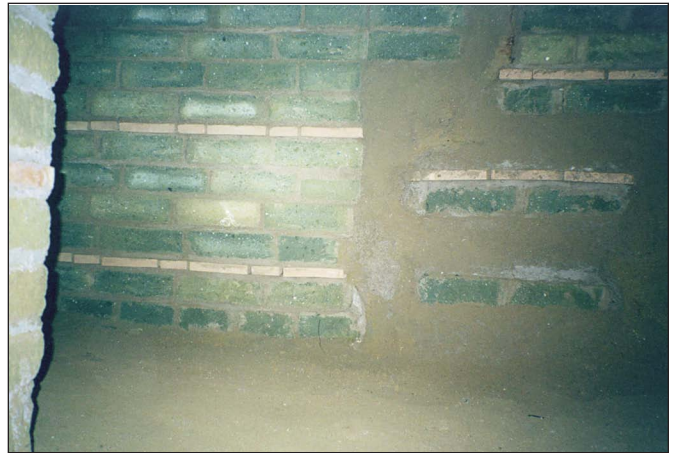
Figure 46. Restored pier in area D. (Photo: J. Dello Russo)
