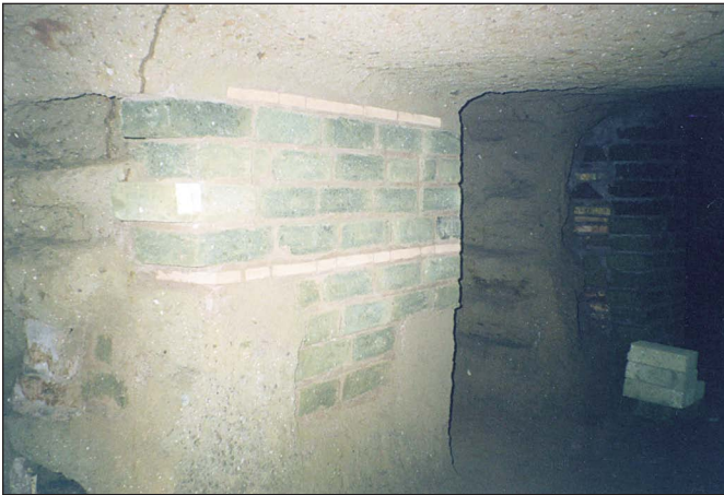
Figure 45. Restored Pier in area D. (Photo: J. Dello Russo)
